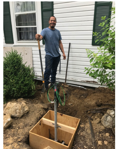
Pablo Ramos installing the new charging station in front of the Main Building
